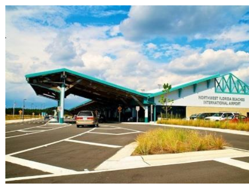
46% Northwest Florida Beaches International Airport
